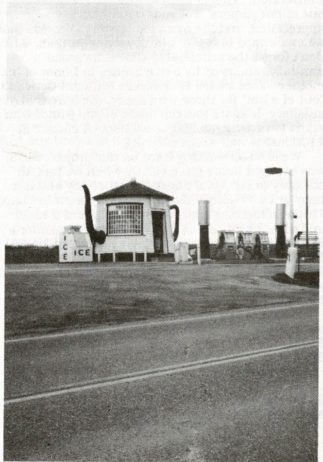
Now a National Historic Site, the Teapot Dome Service Station is located on I-82 several miles southeast of Yakima.
